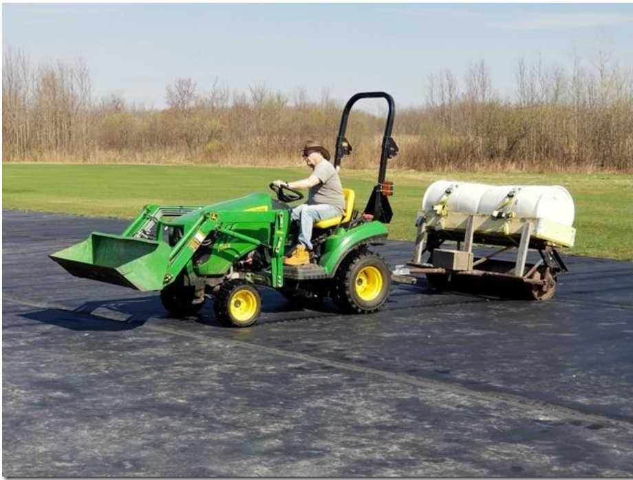
The Geotextile fabric was stretched tight on the ends:
