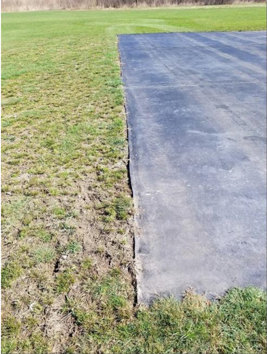
The Geotextile fabric was stretched tight on the ends:
